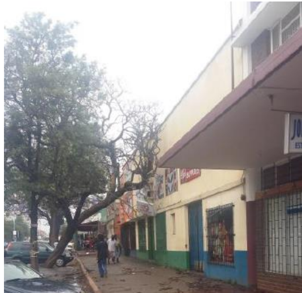
Tree fallen on a building after a storm
