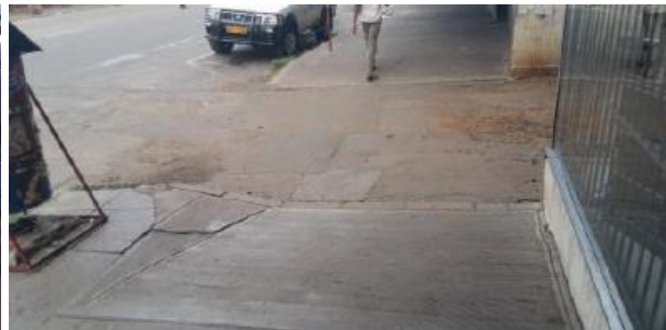
Ramped sidewalk – Service lane interface
