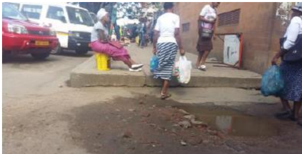
Steep-sided sidewalk – Service lane interface
