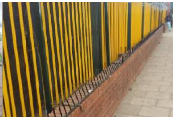
Low wall with spikes, Unity Village
