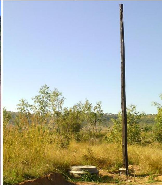
b) Sewer, water and electricity services
