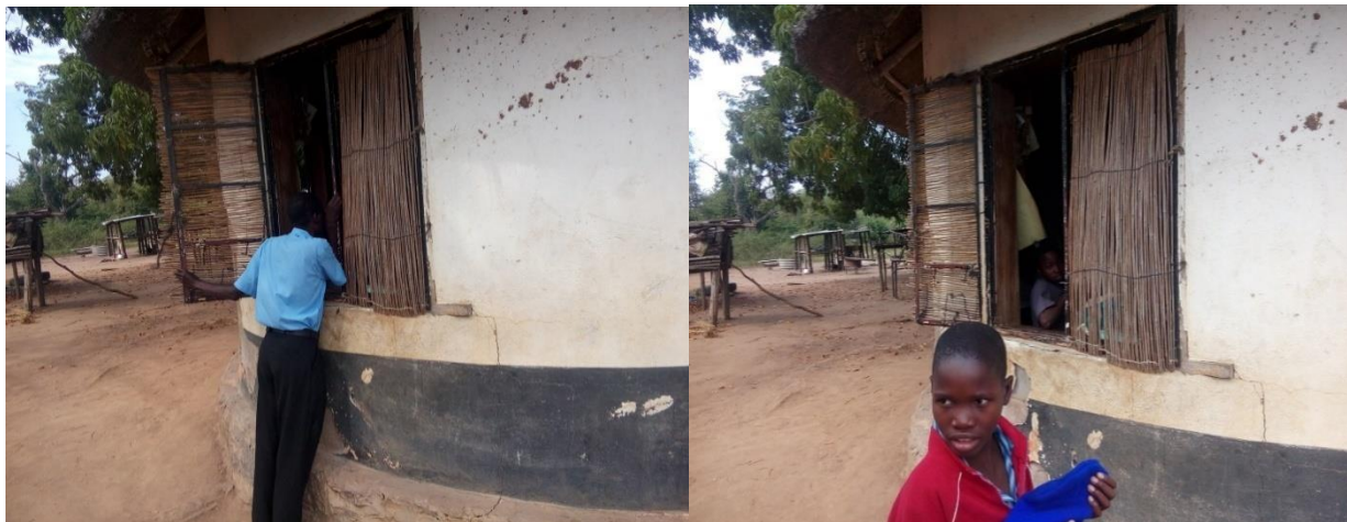
Fig 1: Farm structure converted into primary school classroom. Source: Fbs, (2020)
